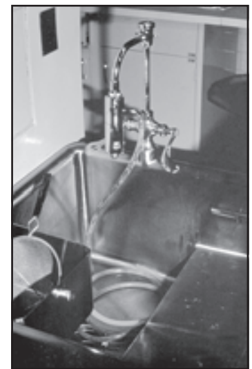
FIGURE 17 Atmospheric vacuum breaker in plumbing supply system
